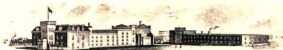
FIREPROOF STORAGE WAREHOUSE
